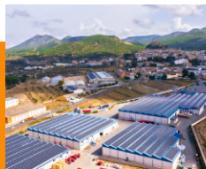
INDUSTRIAL ROOFTOP AISCÁN
