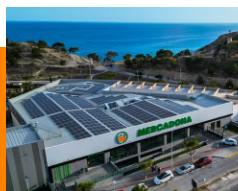
INDUSTRIAL ROOFTOP MERCADONA
