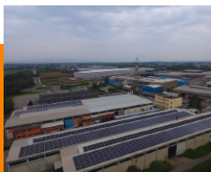
INDUSTRIAL ROOFTOP GAVIOTA SIMBAC
