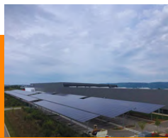
PV CARPORTS KLINE
