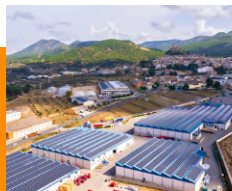
INDUSTRIAL ROOFTOP AISCÁN
