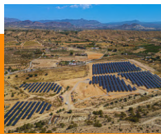
UTILITY SCALE BESIDES
